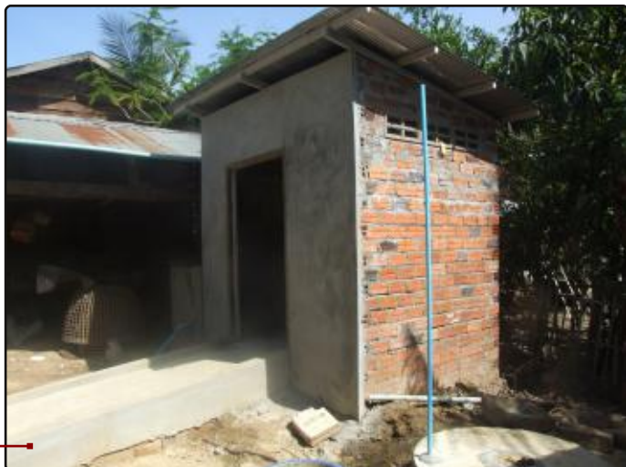
Construction of a toilets in brickwork, work in progress
